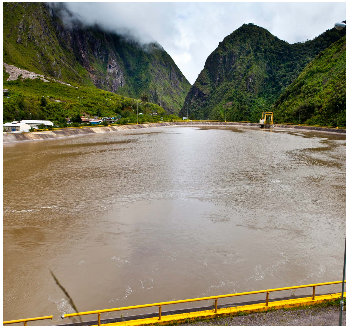
Embalse de Regulación Horaria Central Hidroeléctrica San Gabán II / Horary Regulated Dam of San Gaban II hydroelectric power station
